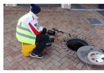
Frogfoot installer deploying FTTH Miniflex through the drains
